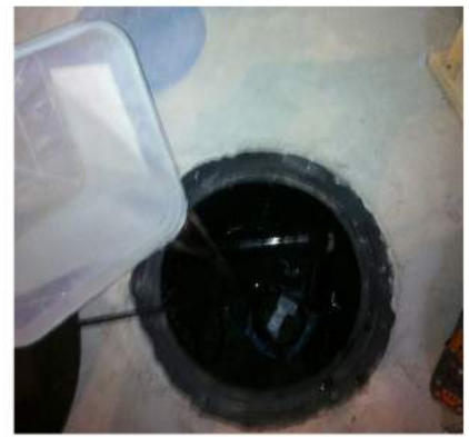
To test sump pump, fill hole with water (by bucket or hose) to about 1 foot above bottom. The round float will rise and when it hits a certain threshold the pump will activate.
